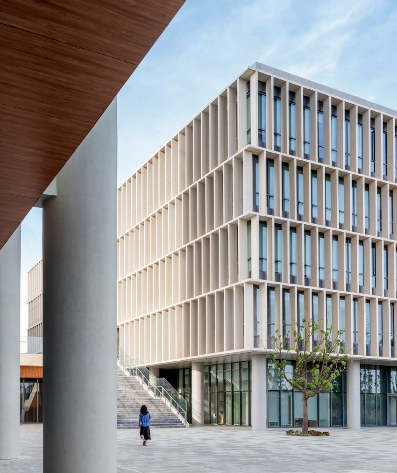
WHITTLE SCHOOL AND STUDIOS, SUZHOU, CHINA | 2 STARS UNDER THE GREEN BUILDING EVALUATION LABEL KNOWN AS CHINA THREE STAR
