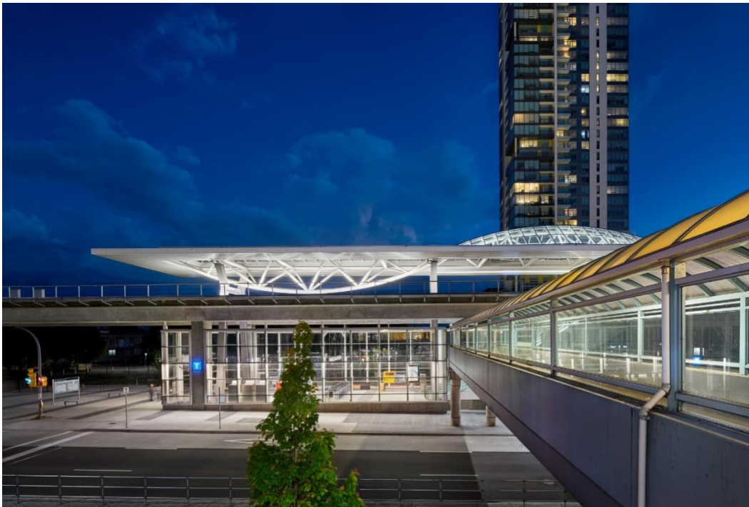
Metrotown SkyTrain Station Renovation in Burnaby, British Columbia, was designed by VIA Architecture. Image courtesy Ed White Photography
